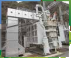
Hydroelectric power plant boost transformers
