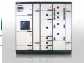
Main LV Switchboard (ATS/STS)
