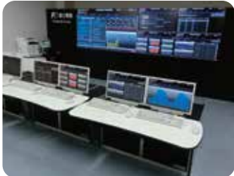
Cluster Energy Management System (CEMS)
