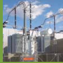
Shunt reactors
