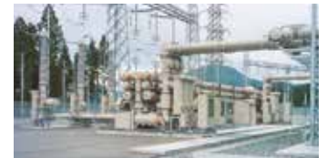
300 kV Phase segregated type gas-insulated switchgears
