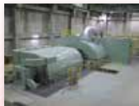
Power generation facilities
