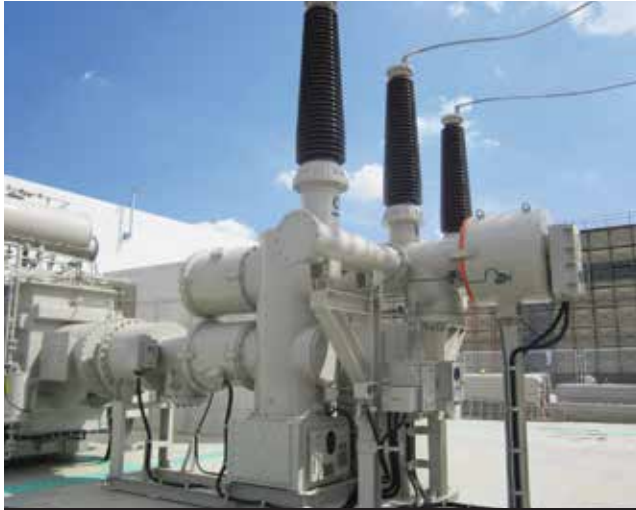
Gas Insulated Switch Gear
