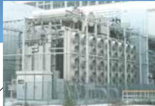
Thermal power plant booster transformers
